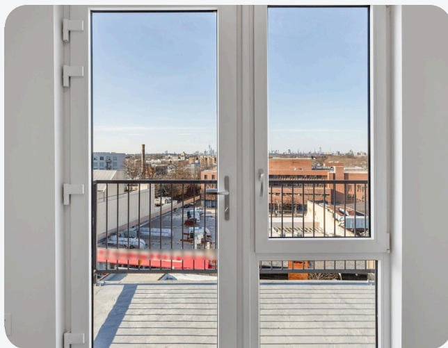
An in-swing terrace door onto a balcony.
