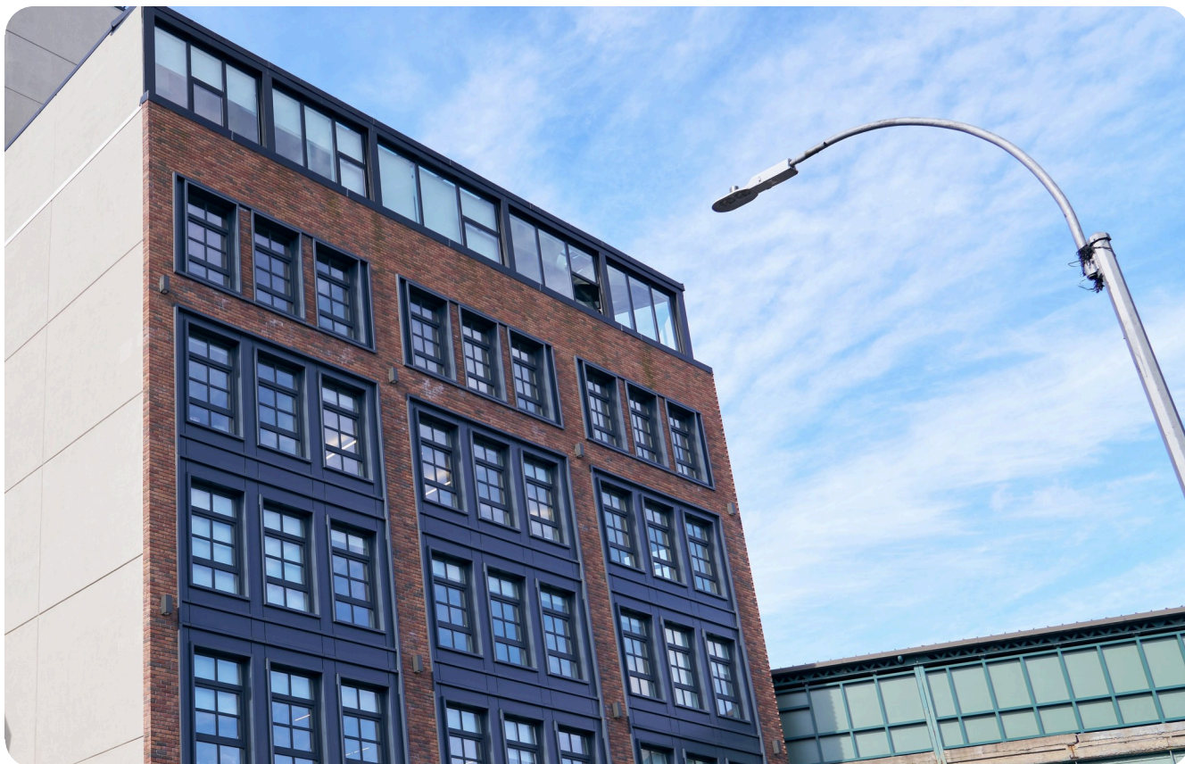
New Utrecht, Brooklyn: Vi6 windows beside an elevated train line.
