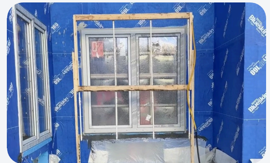
A spray rack set up for a water test on site.
