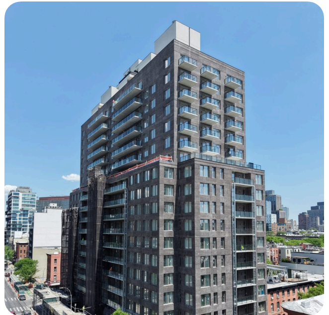
Fourth Avenue Multifamily · Brooklyn
