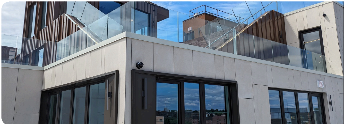
Coney Island, Brooklyn: glazed doors onto a roof terrace, Vi6.
