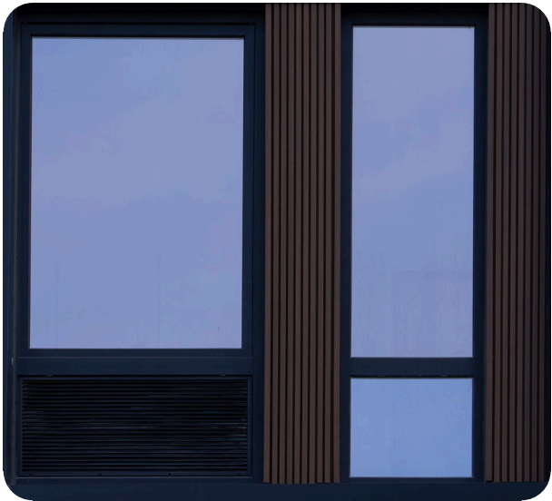
A Parsons window: a fixed lite over a louver in the same black frame.
