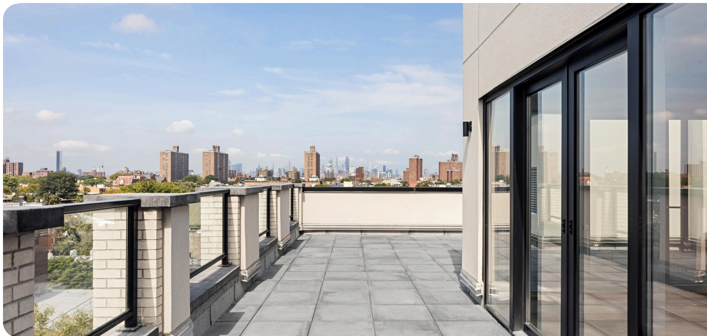
The sliding doors seen from the terrace, black frames against a pale wall.
