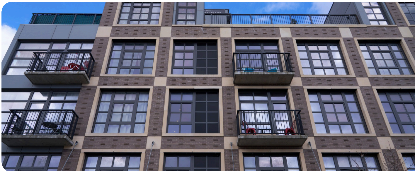
Linden, Brooklyn: Vi6 windows up a brick facade.
